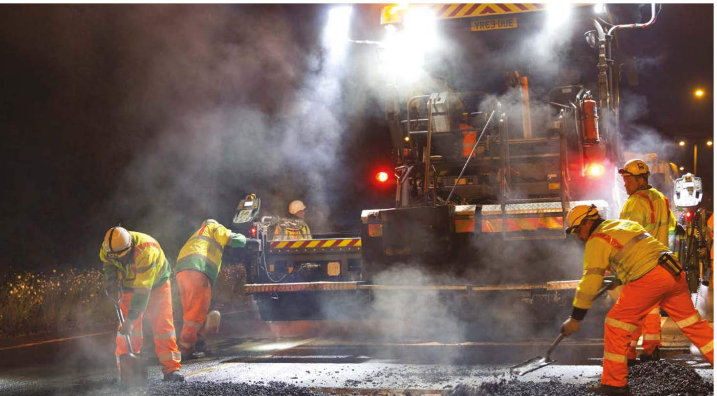
Image courtesy of Highways England.
