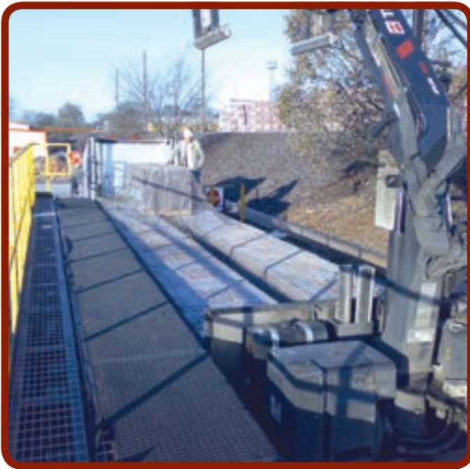
Project: Lorry Netting Station Site: Bishopsbriggs
