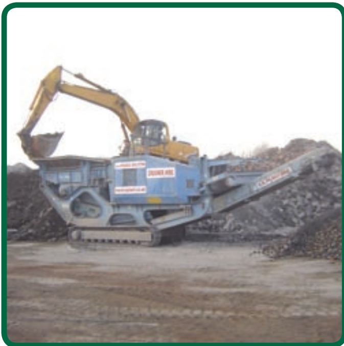
Project: Innovative Use of Recycled Materials Site: Dewsbury
