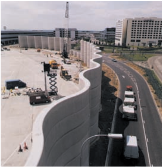
Constructing the wave wall at Gatwick Airport.
