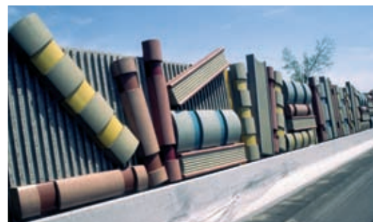
The precast book spines provide a sense of place near a town in central France. The integral concrete safety barrier protects the acoustic barrier from traffic.
