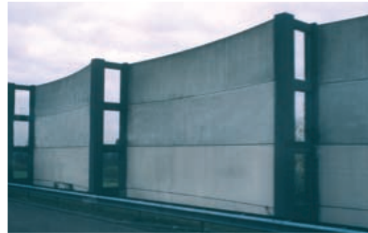
Interest is provided for drivers by a view of the countryside through this staggered acoustic barrier in The Netherlands.
