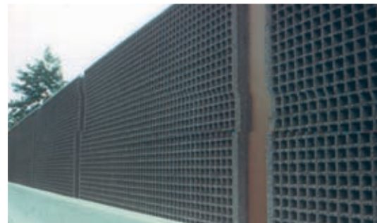
For this barrier, open texture concrete is cast in a honeycomb profile to maximise the sound absorption provided by the surface.
