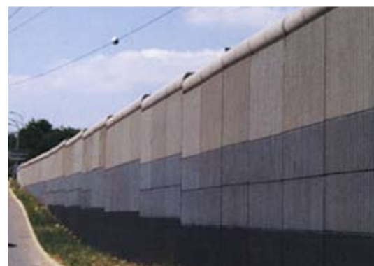
Shades of blue enhance this tall acoustic barrier flanking the A104 south of Paris, which incorporates sound absorbent panels and an anti-diffraction coping.
