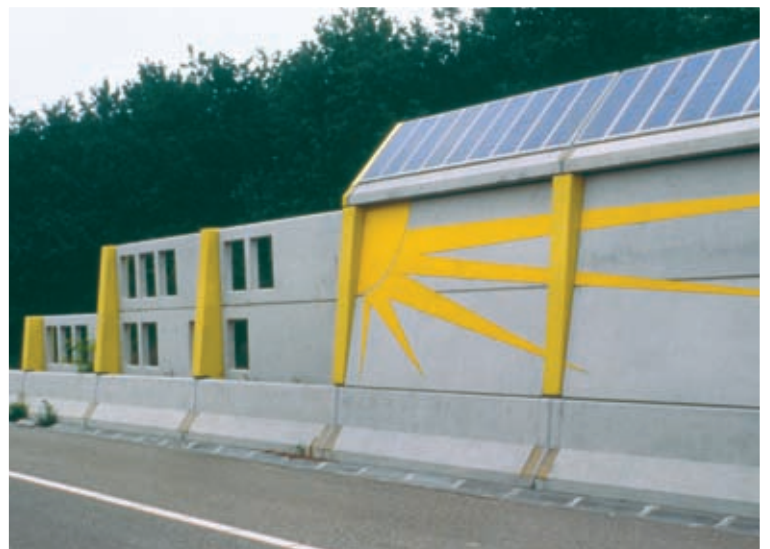
The sunray motif used at the end of this barrier in Utrecht, The Netherlands, signals that the barrier supports solar panels.
