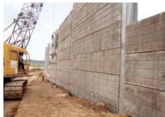
Construction of a precast acoustic barrier.
