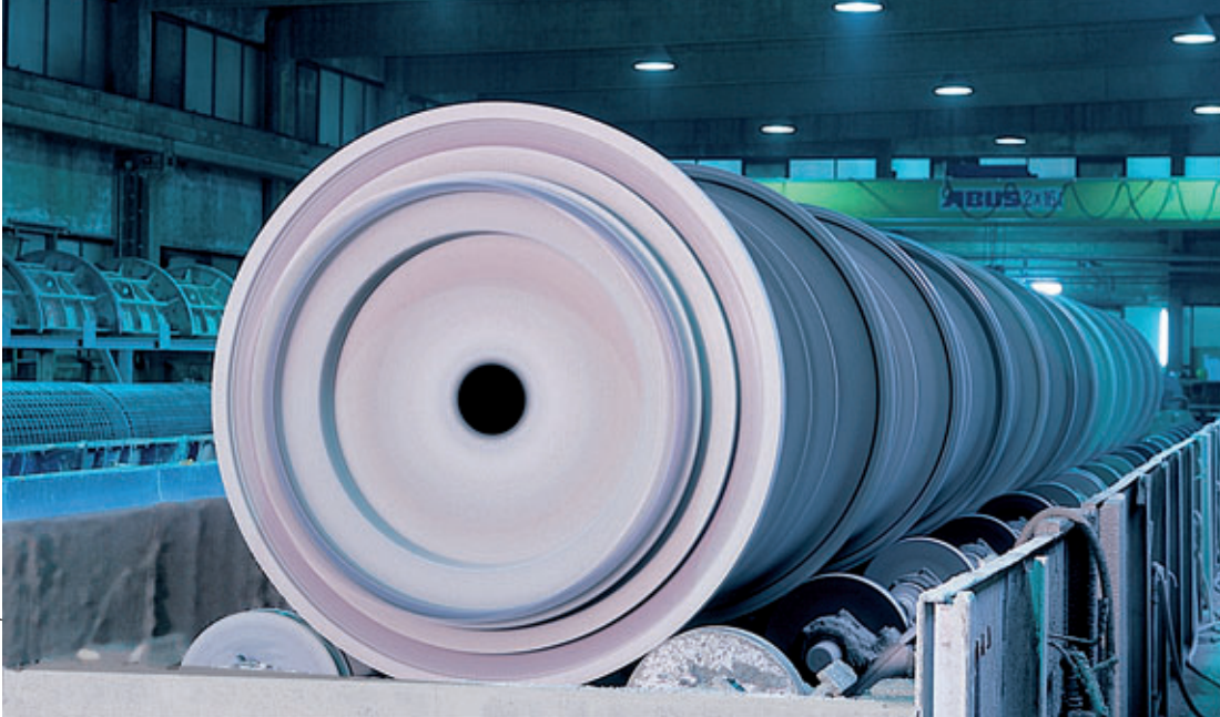
The concrete rotates in the formwork on the spinning machine for about 10 minutes at around 600 rpm
