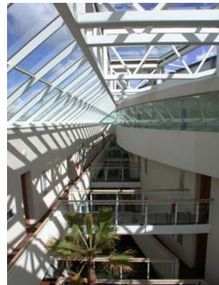
Figure 1e: Energy efficient apartment building in Dublin, Ireland. (Courtesy of Concrete Development Group, Ireland)
