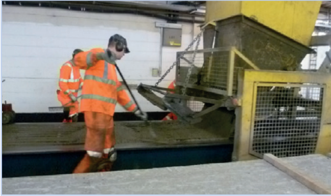
Figure 8.2 Wet casting T-beams.
