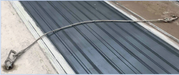
Figure 7.5 Wire restraint secured over hollow core flooring bed.
