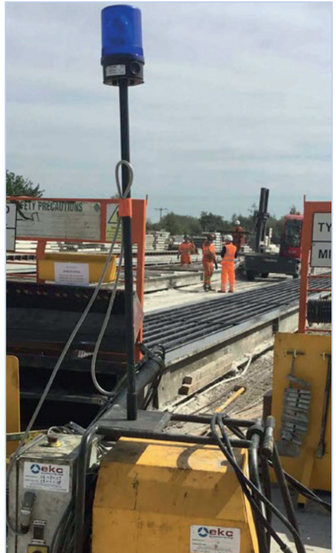
Figure 7.23 Flashing light on mobile stressing unit.
