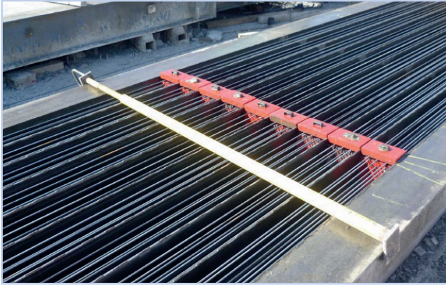
Figure 7.12 Restraint bar placed over T-beam casting bed.
