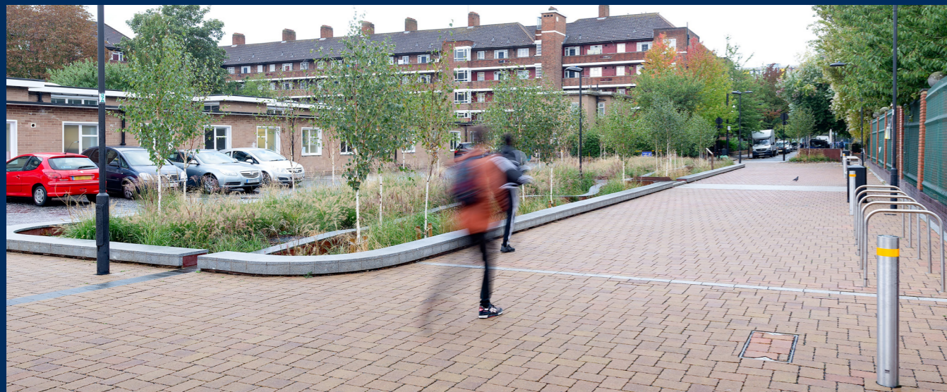
Image | At Bridget Joyce Square, London, a typical, adopted asphalt street and adjacent parking areas were transformed for community use with CBPP overlay shared surfaces and tree-planted raingarden basins – an exemplar for future urban landscapes. Photos: Robert Bray Associates.
