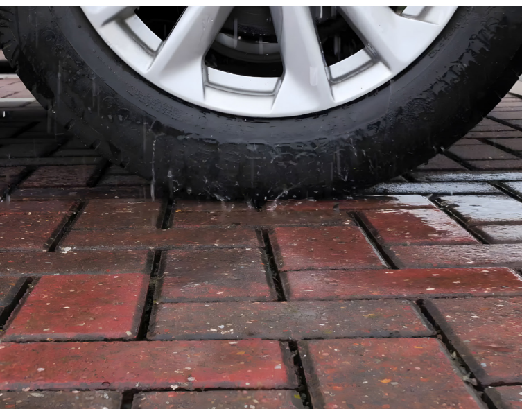
Image below | Rainwater passes straight off CBPP through permeable joints between blocks. Image top right | CBPP avoids the ponding experienced with conventional sealed paving.
