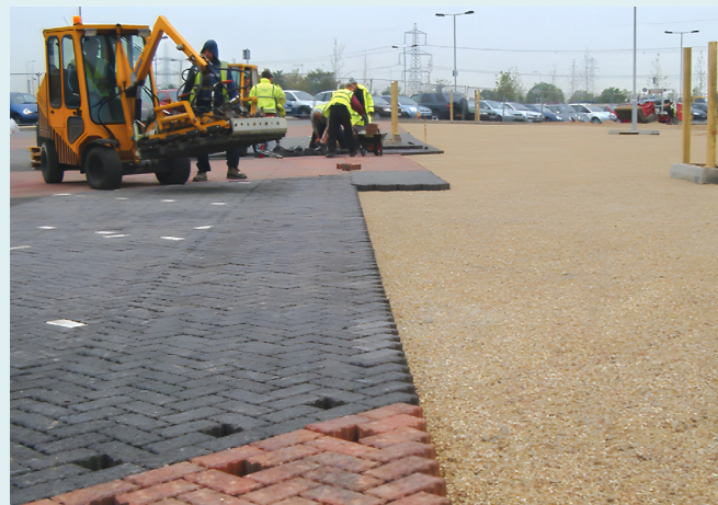
Machine laying of concrete paving units offers a particularly efficient solution for permeable as well as conventional block paving.
