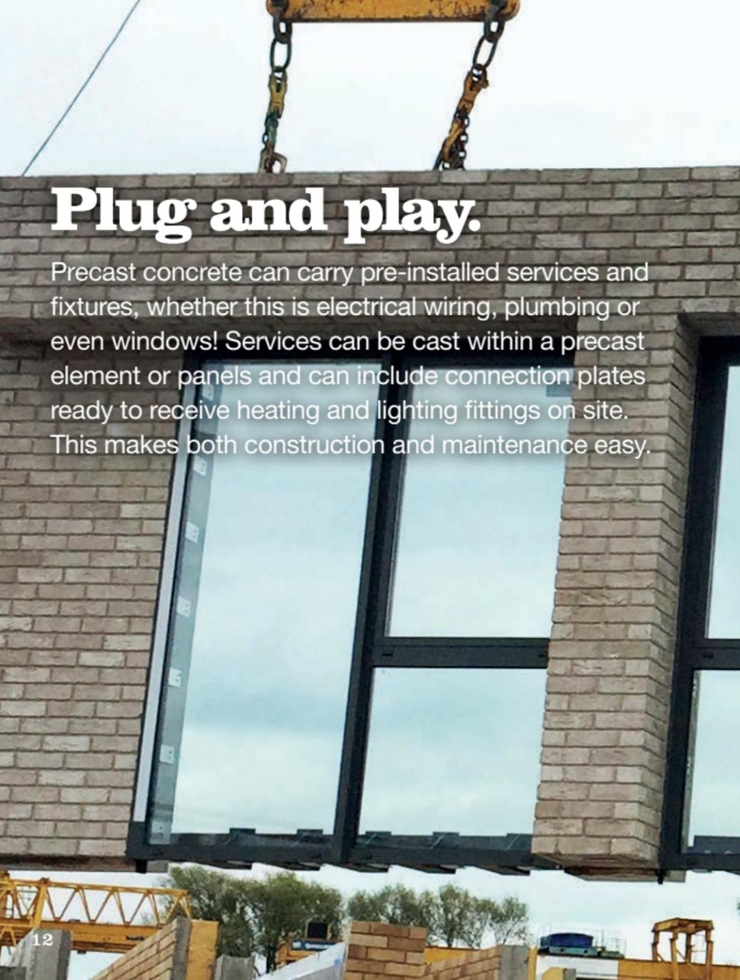
A large precast concrete panel with two windows is being lifted by a crane. The panel has a brick-like texture and is suspended by yellow chains. The background shows a clear sky and some construction equipment at the bottom.
